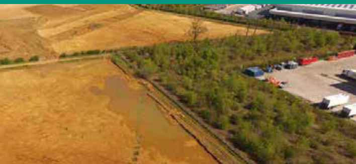
2. Aerial view of the excavation at the site
