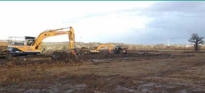
Excavation at the site
